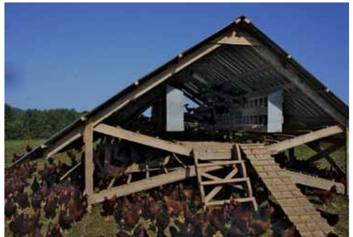
The millenium feathernet uses a catwalk for both human and chicken access to the nest boxes. The A-frame roof design on top of the scissor truss is not only strong, but keeps the birds high and dry.
