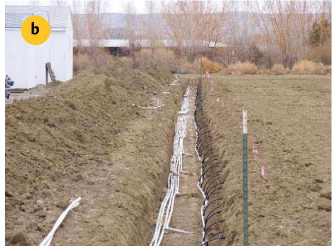
Figure 3. (a) GPS mounted variable rate sprinkler irrigation system and (b) sub-surface drip irrigation system at Powell Research and Extension Center can apply less water than furrow flood irrigation systems while meeting the crop water needs.
